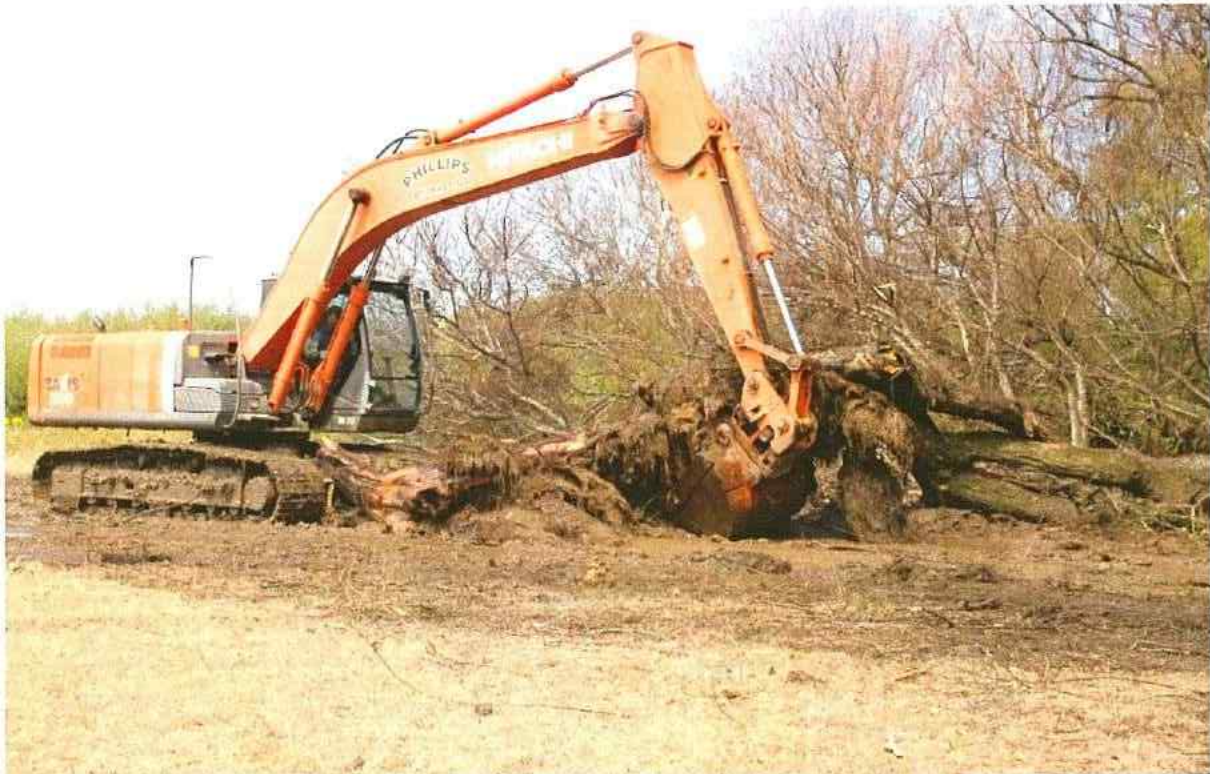
Whitebait Project Papatotara: Prior to building the dams the crack willow (sprayed in October 2018) in the vicinity of the dam sites and along the upstream shoreline of the new Terrace Creek wetland were removed, where practical.
