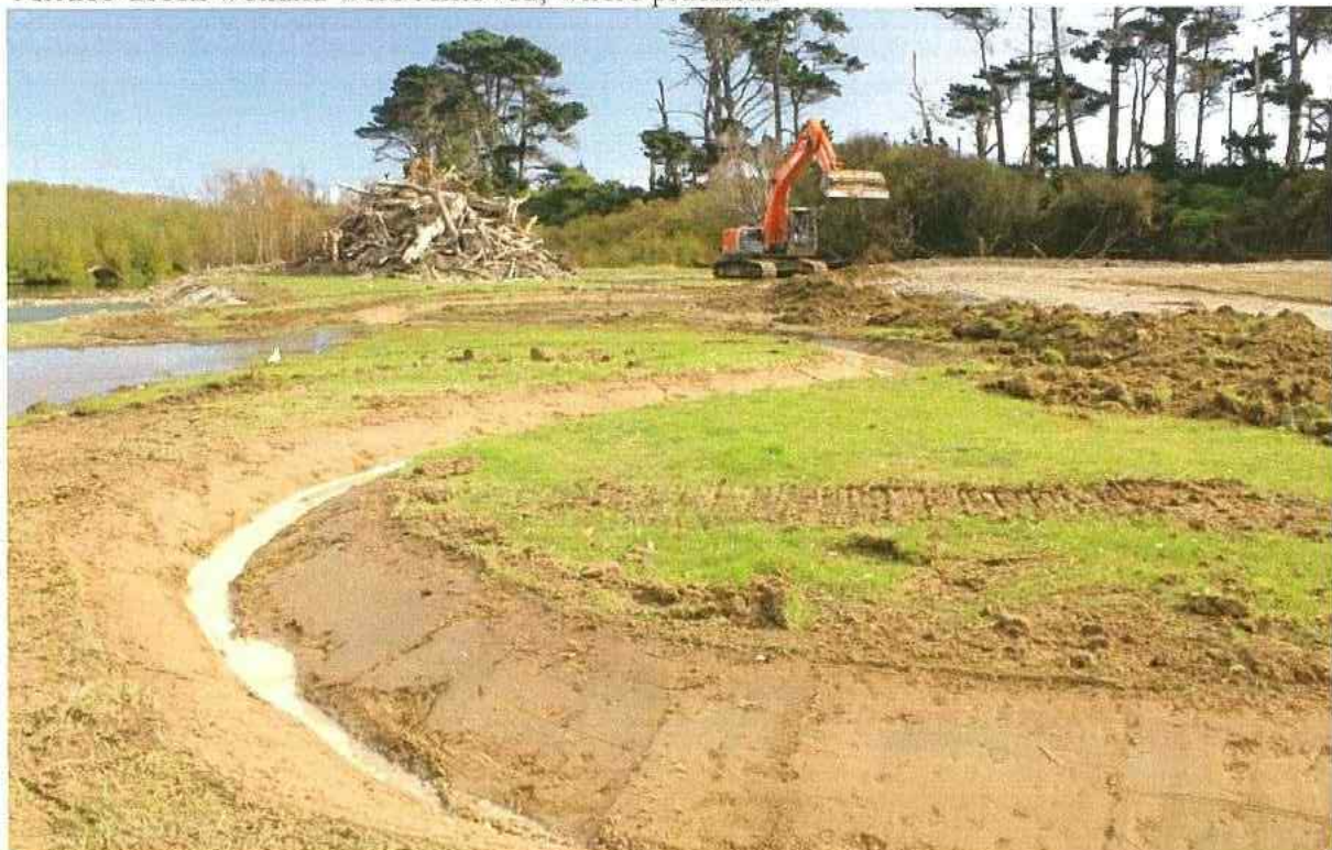
Whitebait Project Papatotara: This photo captures several aspects of the wetland construction job. The digger is placing material on the batters of the Terrace Creek dam in preparation for sowing grass seed. The permanent outlet channel for the Terrace Creek Wetland is in the foreground. To the left, the borrow pit can be seen. It is now new additional habitat and is connected to the Blue Hole (top left of the photo).
