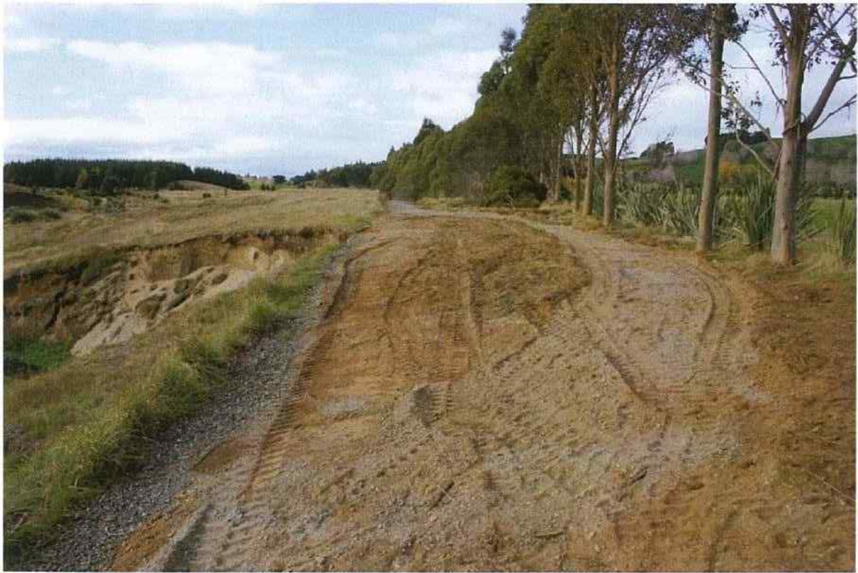
Home Creek Project: Walking track realignment and bank repair work was carried out in April 2018. This work resolved the health and safety issue resulting from flood damage to Home Creek banks in February 2018.
