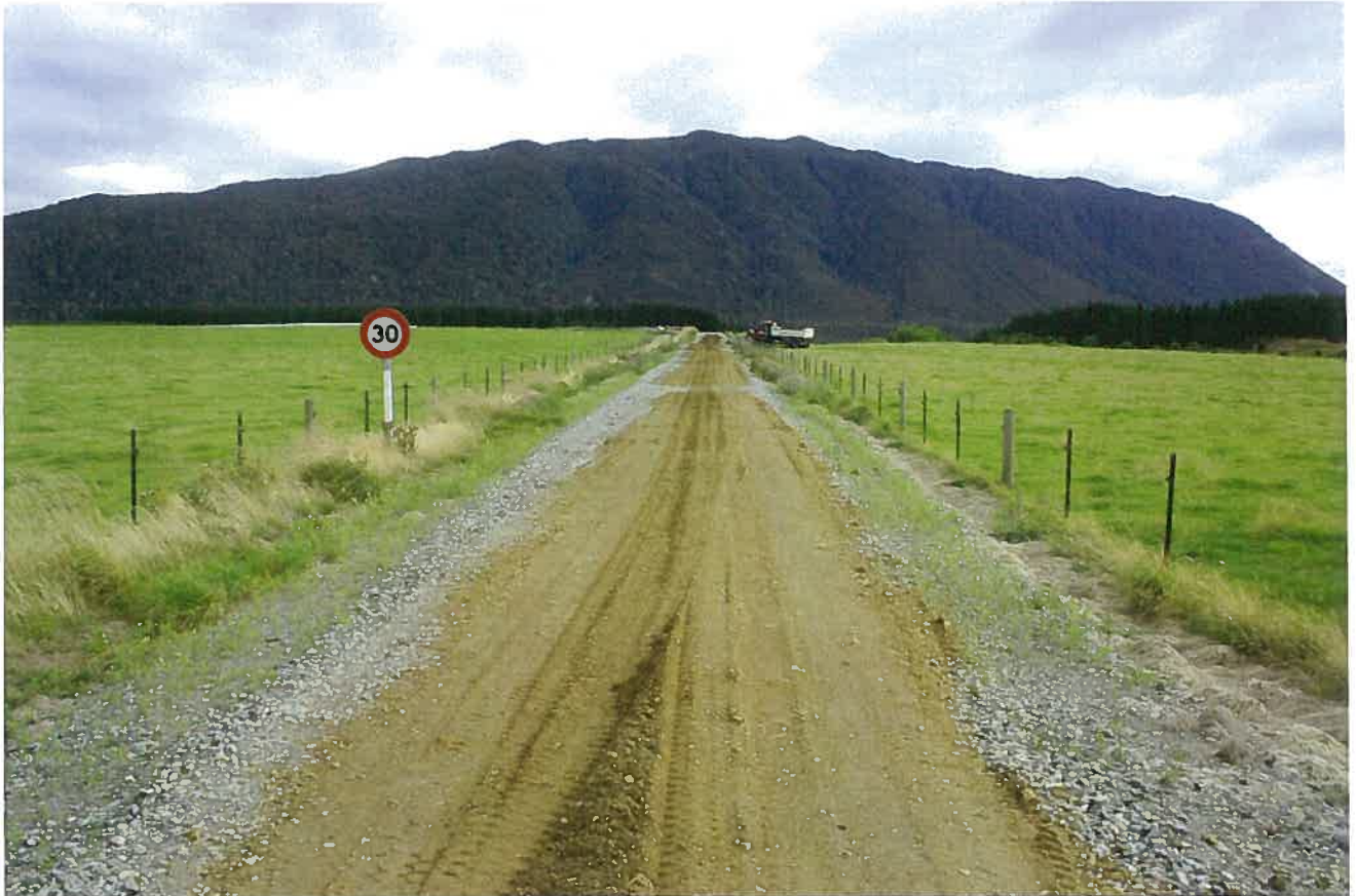
Rakatu Wetlands – access road repairs occurred this year, with more road metal needed and an extra cattle stop (below) being installed. This was the first major maintenance work carried out on the access road in the ten years since the wetlands have been open to the public.
