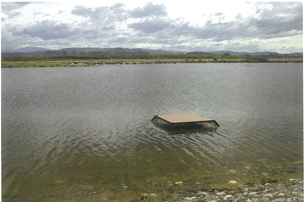
Whitebait Project. The intake siphon is now operational. The installation of the pipes from the siphon, under the bed of the Hollyburn and discharging into the Whitehead Suite of wetlands, was completed in January 2016. Minor adjustments may still be required to maximise benefits of the system.
