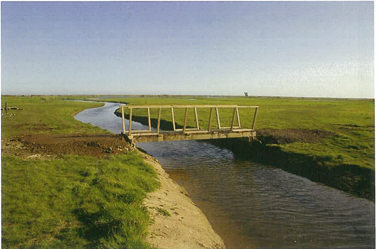
Whitebait Project. Foot bridges, which were surplus to DOC's requirements, have been installed (September 2015) to enable easier foot access around the wetland network. The pictured bridge crosses the Inder diversion channel.
